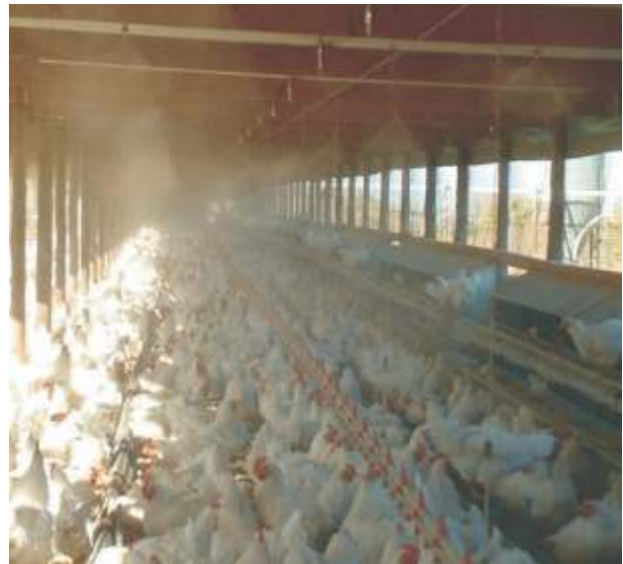
Permanent misting/fogging system in poultry house to reduce airborne contamination
